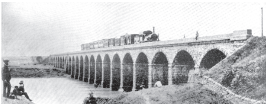
Fig. 1.4 First Railway Bridge linking Bombay with Thane, 1854
